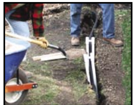
Hold Multi-Flow in the center of the trench while backfilling.
