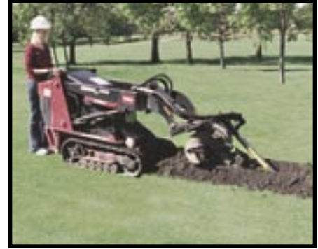
Begin trenching at the lowest point and proceed up grade. Always check with local utilities before digging.
