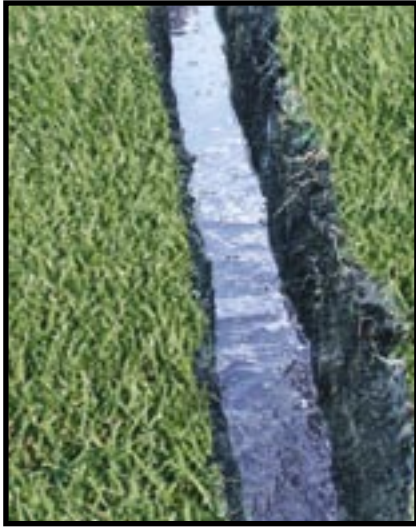
The open trench is the most basic model for an artificial drainage system.
