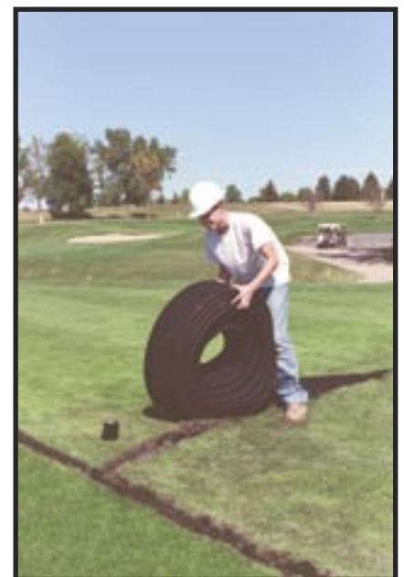
Roll out the pipe beside the trench and lower it into place. Use Multi-Flow connectors to ensure a secure transition between lines.
