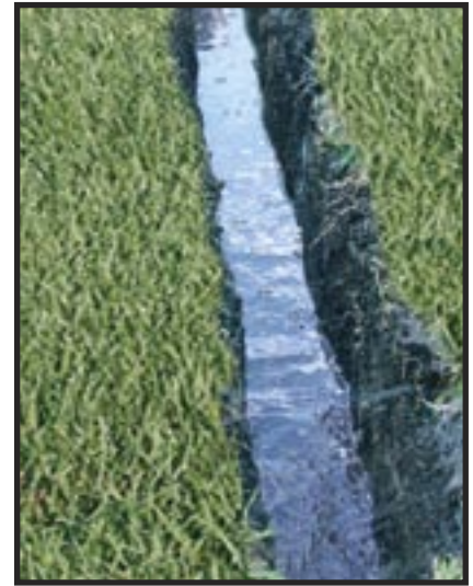
The open trench is the most basic model for an artificial drainage system.
